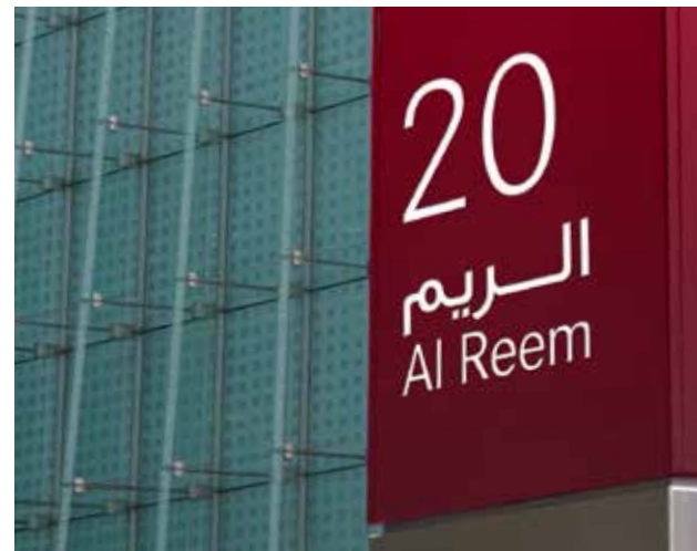
Aluminium monolith powder-coated with white vinyl graphics
